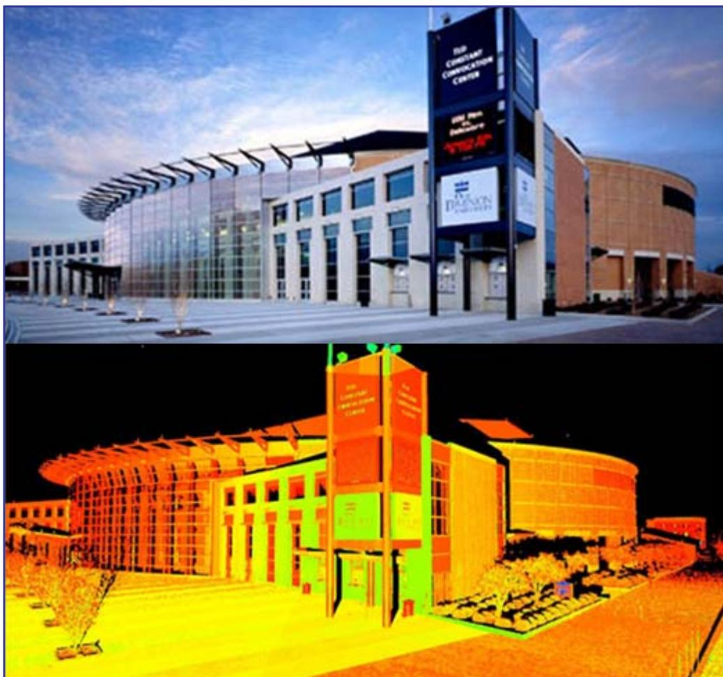
Figures 1&2: The Constant Convention Center at ODU (above) and an image produced from a 3D Laser Scan of the Constant Convention Center (Image and 3D Laser Scan courtesy of Brian Daniel and Loyola Spatial Systems).
